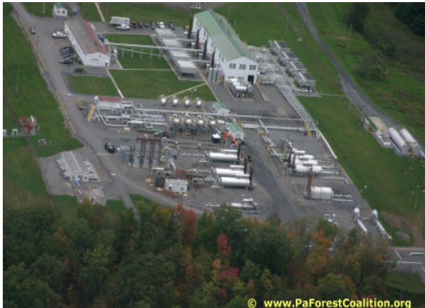
Compressor Station in the Susquehannock State Forest
